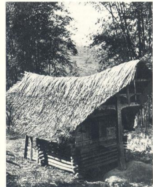
32. An old-fashioned Toraja house with crossed-log foundation structure in Sareale district, Tana Toraja, 1982. (Photograph: Roxana Waterson)
